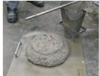
Test trials on PFAC at Island Concrete Batching Plant, Singapore
