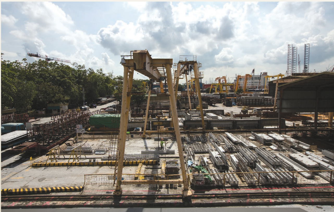
A precast concrete facility of Hong Leong Building Materials Group in Singapore.
